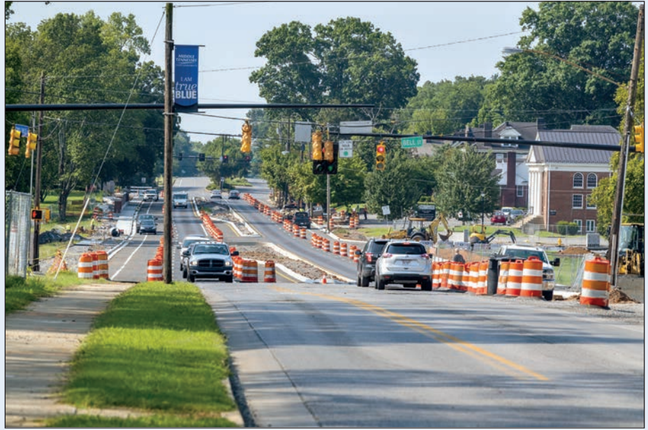
The Middle Tennessee Boulevard construction project has reached the halfway point.
